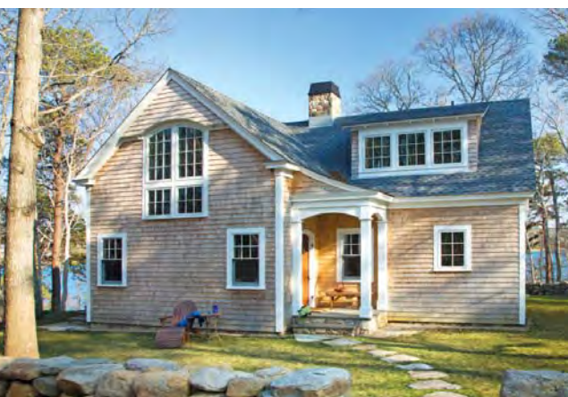
The exterior of the Tashmo Cottage is covered in white cedar shingles, which eventually will turn a beautiful gray, weathered-wood tone from exposure to the salt air. The home sits amid the trees with views of the lake, an ideal refuge.
